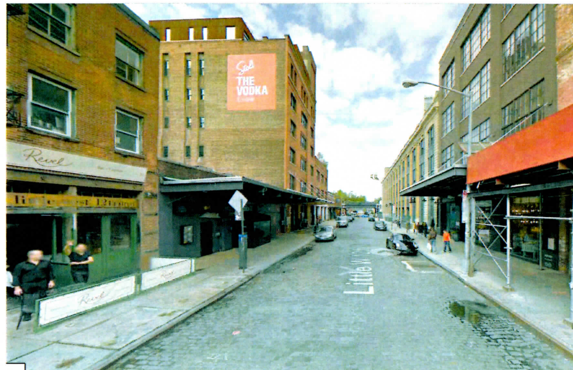
PREVIOUSLY INSTALLED PAINTED NON-ILLUMINATED SIGN
